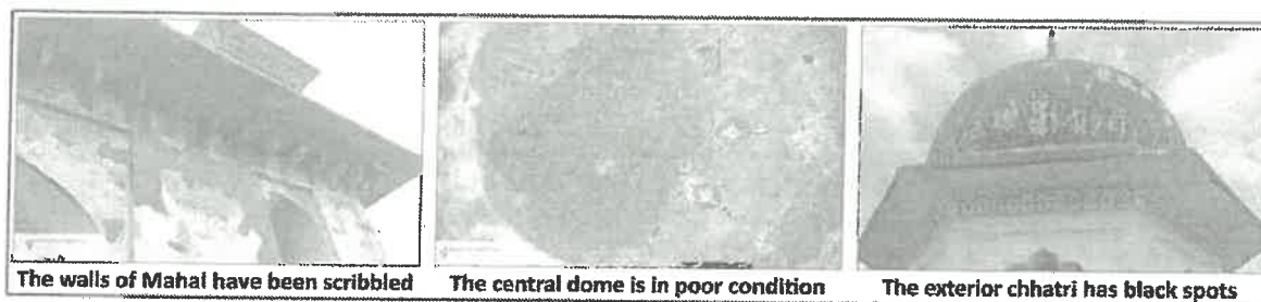
Figure 26: Present Condition of the Structure
