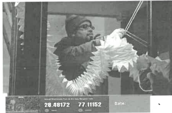
Installation of the project
