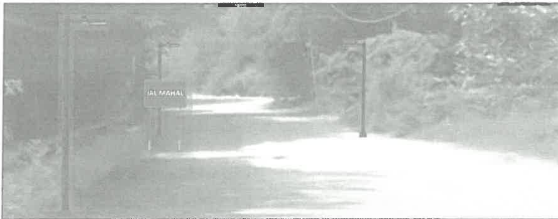
Figure 19: Installation of Signages and Street Lights on the Approach Road
