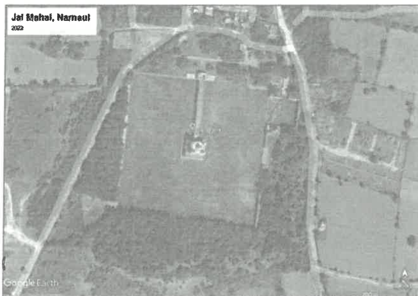
Figure 10: Present Condition of Jal Mahal, Narnaul Source: Irrigation Department, Narnaul, 2022
