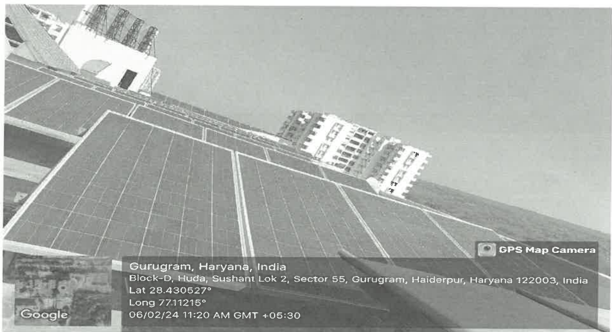
Solar panel installed on the roof top of D Block building
