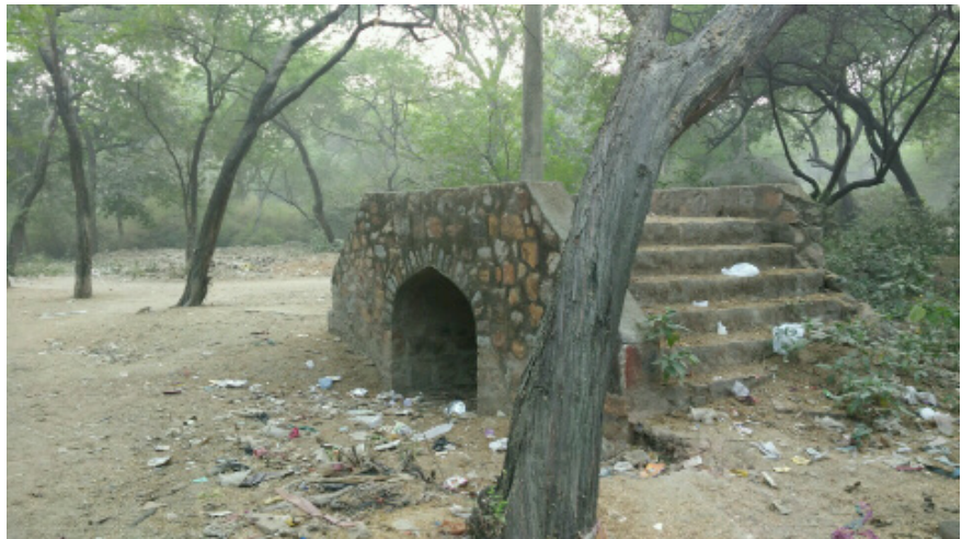
Figure 5: Drainage Structure enroute Rajon ki Baoli (Source: Author)
