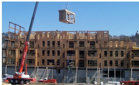
Figure 2: Example of prefabricated construction in process. (Source: Free photograph on Pixabay)
