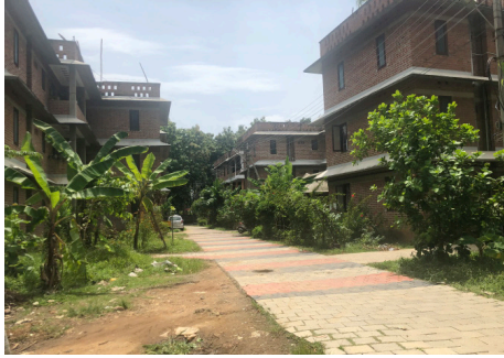
Figure 4: Kalladimukham Colony, Redevelopment Project in Kerala (Source: Author)
