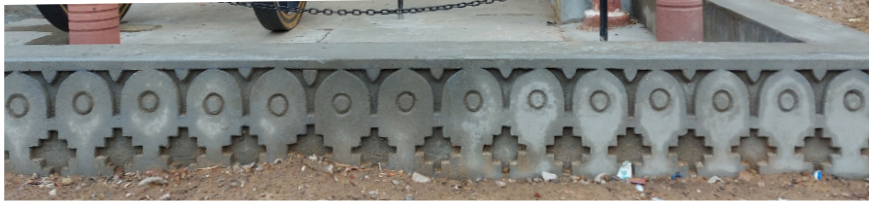
Figure 2: Cement carving work (Source: Author)
